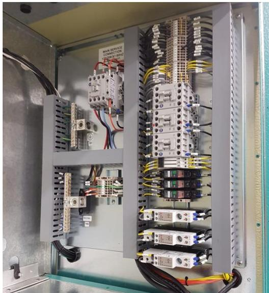
Figure 2-11 Electrical Service Line Connections
