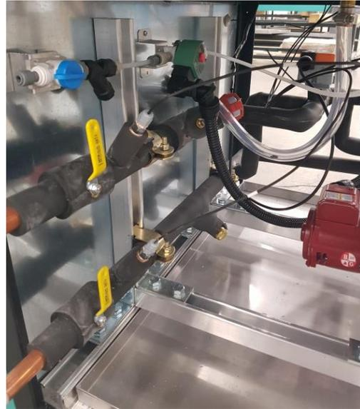
Figure 2-7 Glycol Cooled System Connections
