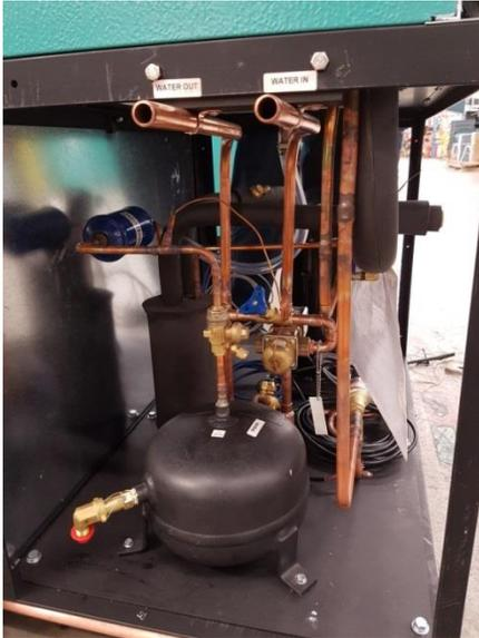
Figure 2-6 Water Cooled System Connections
